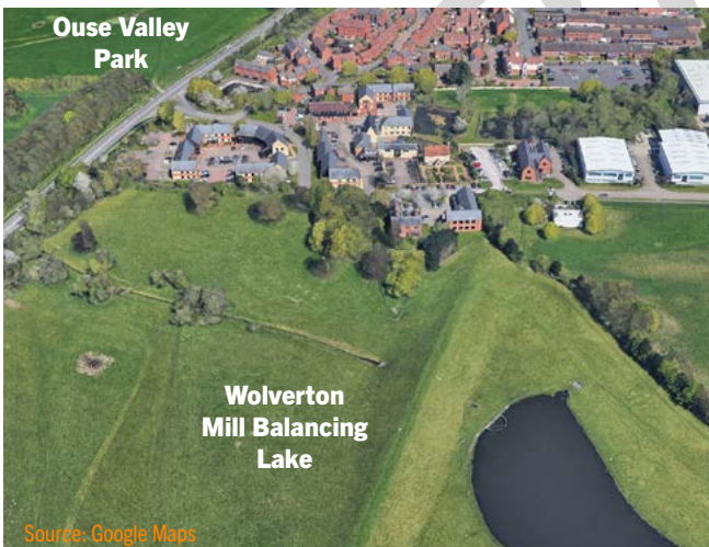
Figure 28 Wolverton Mill Business Park has office buildings adjacent to and overlooking adjoining parkland
