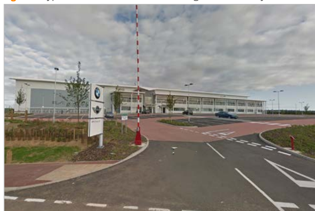
Figure 6 Typical distribution Centre building in Swan Valley
